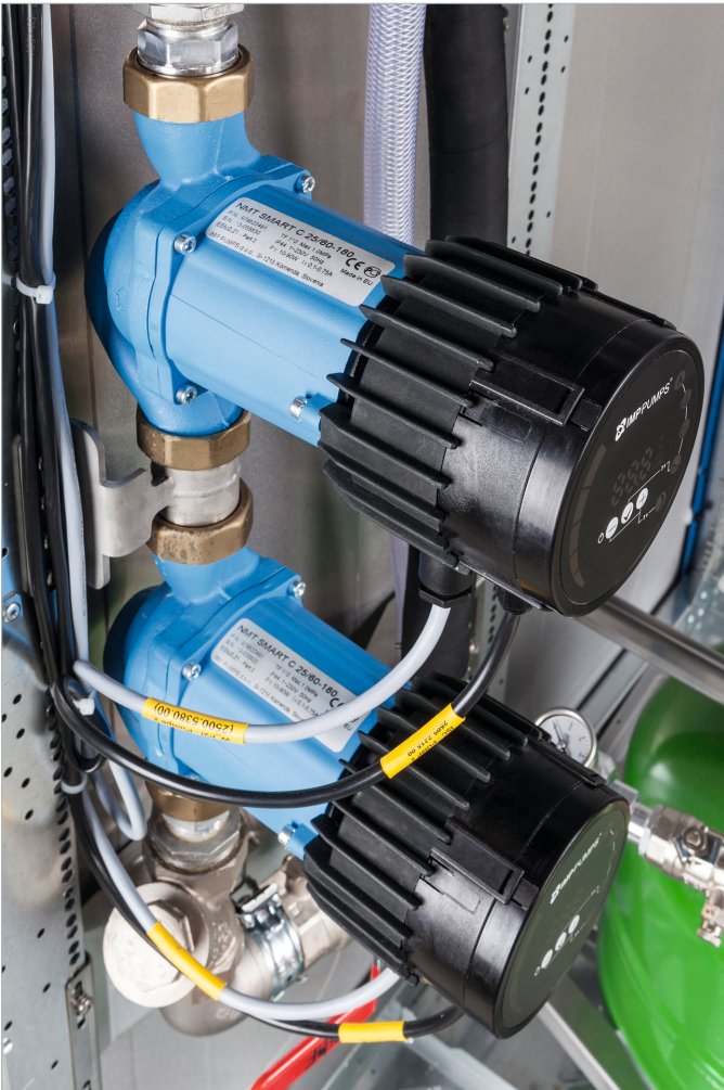
Compact cooling system with redundant pump modules
